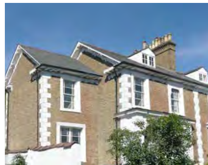
Community: Best practice photograph A similar architectural approach is continued in this side extension by Sam Causer
