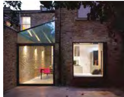
An angled glazing providing daylight to the extension without overshadowing the neighbor by Platform 5 Architect
